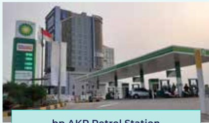
bp AKR Petrol Station
